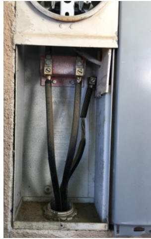
Figure 13 – Inside of PG&E Cable Termination Compartment - Picture Set 4
