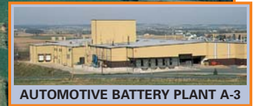
AUTOMOTIVE BATTERY PLANT A-3
