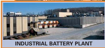
INDUSTRIAL BATTERY PLANT
