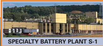
SPECIALTY BATTERY PLANT S-1
