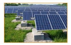
This is a common foundation method especially for brownfield sites, such as landfills, where there is a cap layer that cannot be penetrated. Ballast foundations can be either cast-in-place or pre-cast depending on project requirements and shipping costs.
